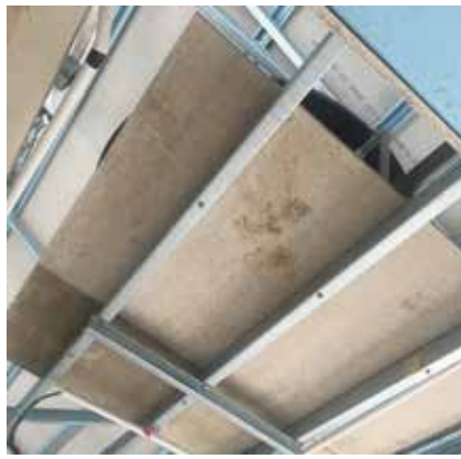
PRIMA C-Studs to support water tank
