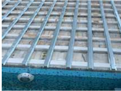
PRIMA Tophat framing for decking system
