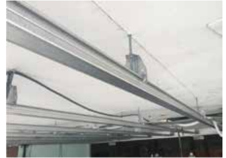
PRIMA Flipped Direct Fixing Clips
