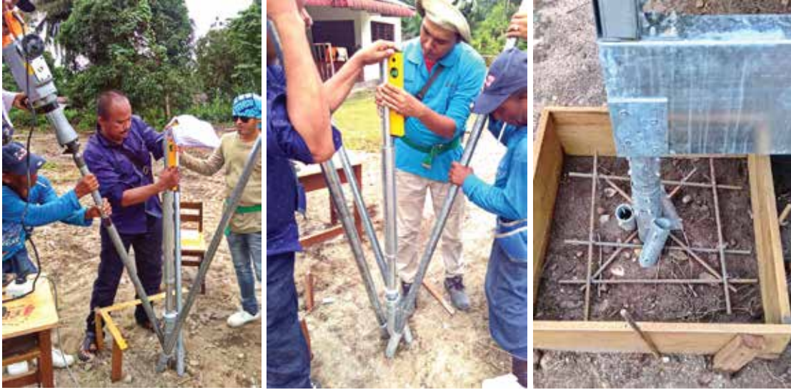
Tri-pod concept of soil anchoring
