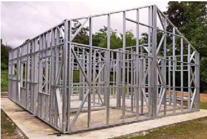
LGS Frames Structure
