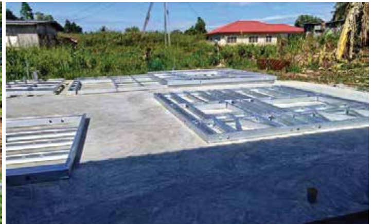
LGS frames at site ready to install
