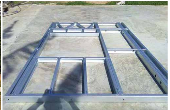
LGS Frame before installation
