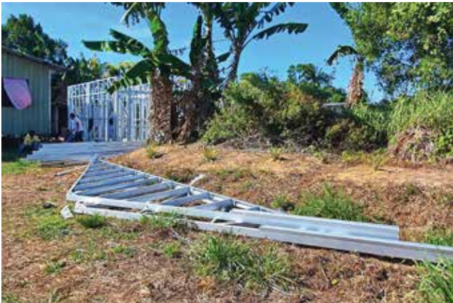
LGS frames at site
