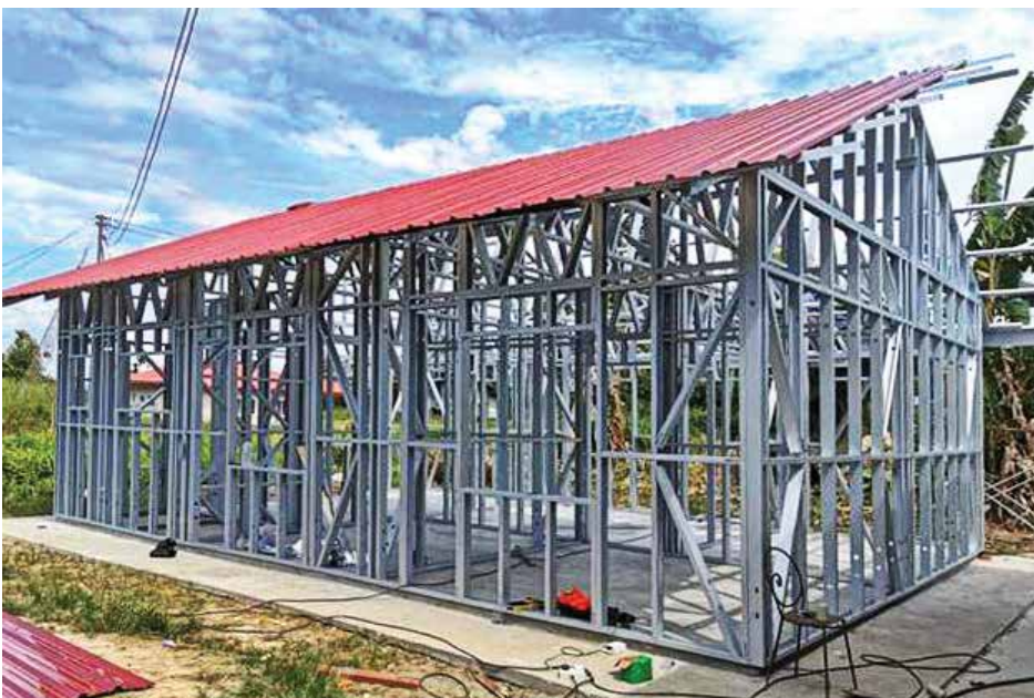
Roof installed on LGS frames to protect working area
