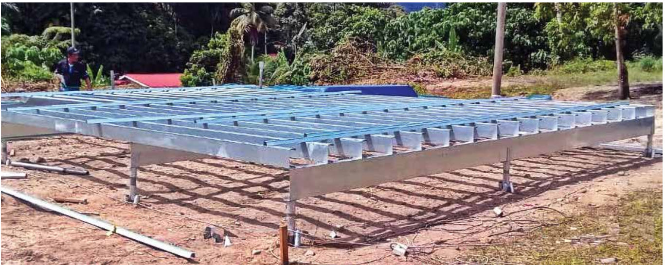
IBS Proprietary Anchorage System for elevated house
