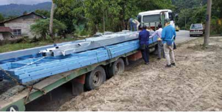
LGS frames deliver to site in bundle
