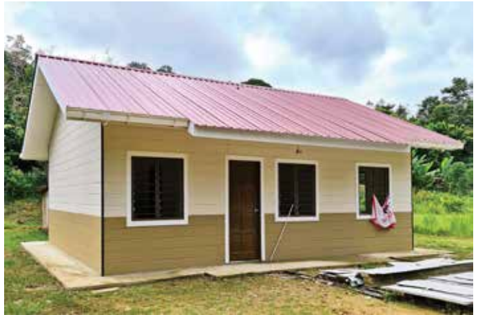
PPRT Kampung Ibol, Sri Aman, Sarawak, Malaysia Size : 660 ft 2 Consist of 3 bedrooms, living room, dining area, kitchen, 1 bathroom and 1 toilet
