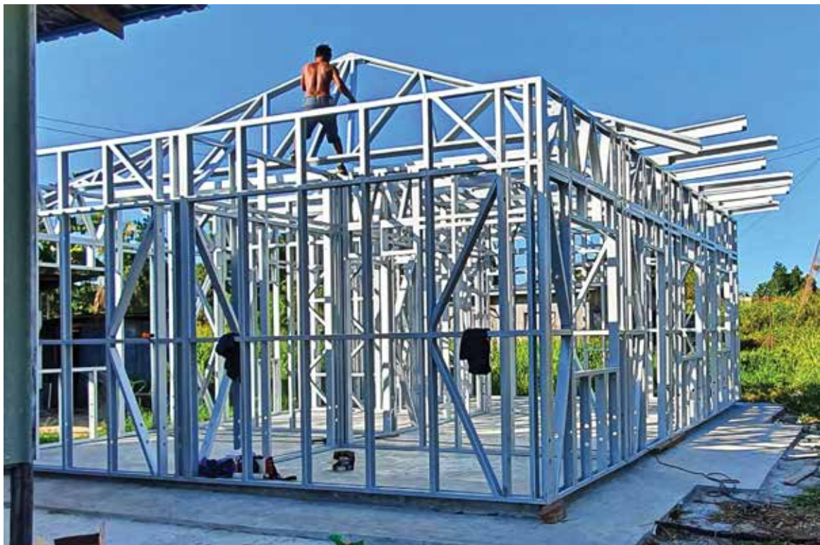
LGS frames installation for landed house on RC Slab foundation
