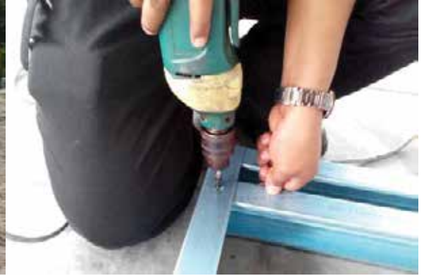
LGS frame installation using electric drill
