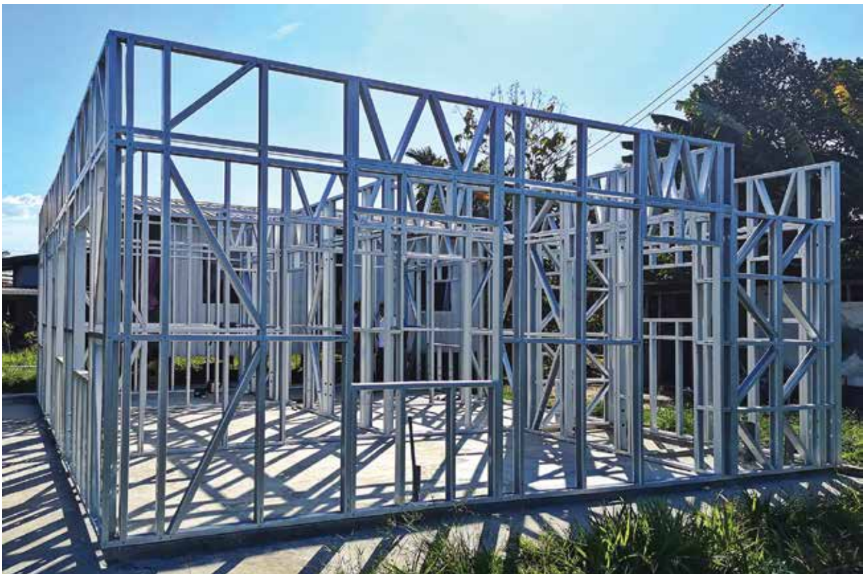
LGS Frames Structure
