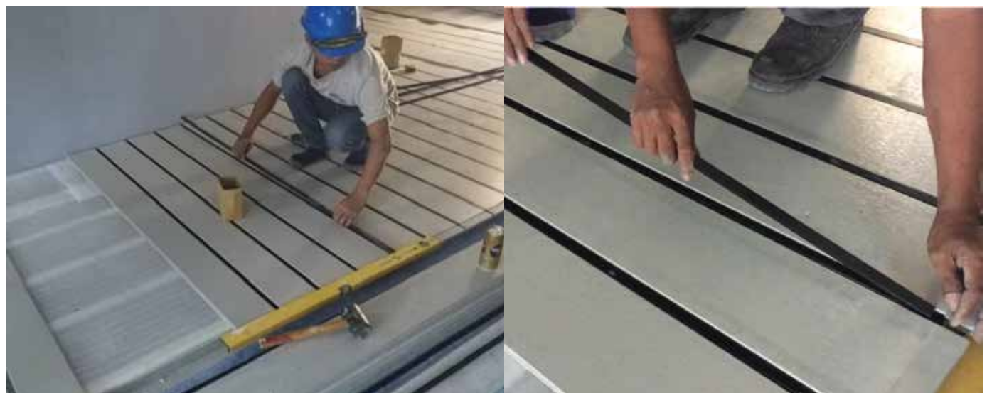
Figure 3 : Install the PRIMA Decking CFS (Top Cover) to conceal the fasteners (Snap-on method).
