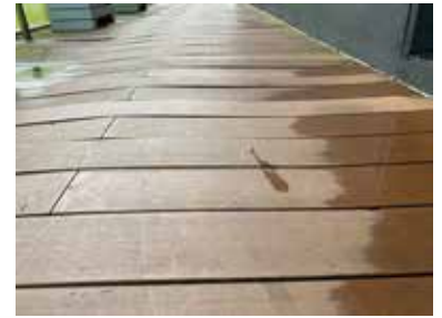
Wood Plastic Composite (WPC) decking, tendency to warp after exposed to heat & rain.
