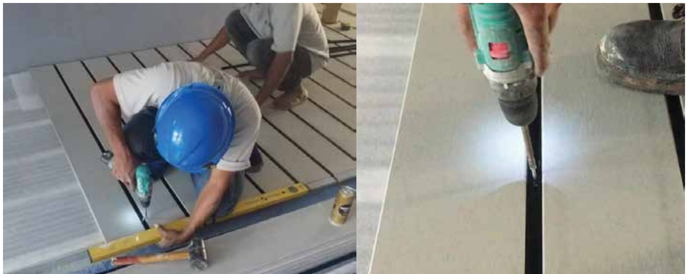
Figure 2 : Fasten the PRIMA Decking CFS (Base Unit) to framing joist using PRIMA Fastener .
