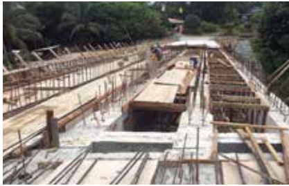
Conventional method requires various propping to support the concrete pour
