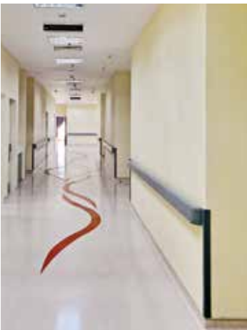
Crash Rail installed on PRIMA drywall
